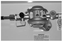
Your caravan is supplied with a wall mounted gas regulator plumbed inside the gas cylinder compartment. The regulator and all appliances work at a harmonised 30mb pressure, which work with Butane and Propane gas.
