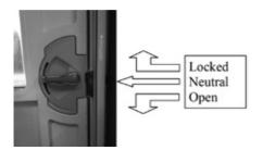
The door flyscreen is tracked top and bottom and operation must be by the centre of the handle to aide a smooth operation.
