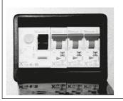
Black lever switch, far left – Residual Current protection Device (RCD) and main 230V on / off switch.
