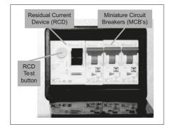
The Residual Current Device (RCD) is basically provided to protect the user from lethal electric shock. The RCD will turn off (trip) if the current flowing in the live conductor does not fully return down the neutral conductor, i.e. some current is passing through a person down to earth or through a faulty appliance.
