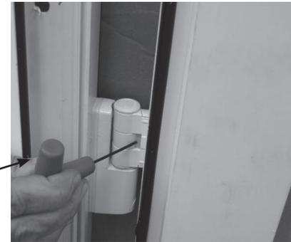
To adjust the door vent horizontally (left to right). Open the door and push in the plastic clip.
