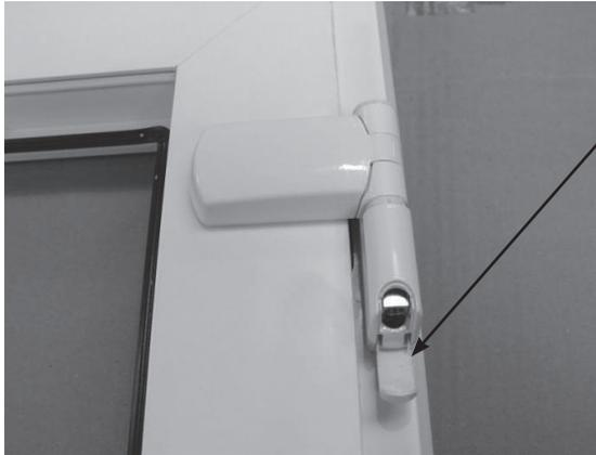
To adjust the door vent compression and height within the frame unclip the cap as shown.
