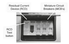
The Residual Current Device (RCD) is basically provided to protect the user from lethal electric shock. The RCD will turn off (trip) if the current flowing in the live conductor does not fully return down the neutral conductor, i.e. some current is passing through a person down to earth or through a faulty appliance. To ensure the RCD is working correctly, the test button should be operated each
