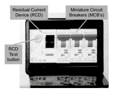
The Residual Current Device (RCD) is basically provided to protect the user from lethal electric shock. The RCD will turn off (trip) if the current flowing in the live conductor does not fully return down the neutral conductor, i.e. some current is passing through a person down to earth or through a faulty appliance.
