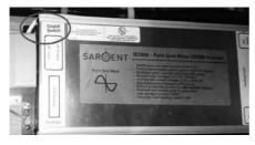
If no other source is available, the inverter will supply 230v power to the sockets in the appropriate list above, converting 12v power from the leisure batteries into 230v power at the sockets.
