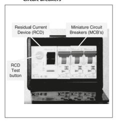
The Residual Current Device (RCD) is basically provided to protect the user from lethal electric shock. The RCD will turn off (trip) if the current flowing in the live conductor does not fully return down the neutral conductor, i.e. some current is passing through a person down to earth or through a faulty appliance.
