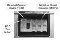
The Residual Current Device (RCD) is basically provided to protect the user from lethal electric shock. The RCD will turn off (trip) if the current flowing in the live conductor does not fully return down the neutral conductor, i.e. some current is passing through a person down to earth or through a faulty appliance.
