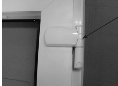
Hinge in the supplied position
