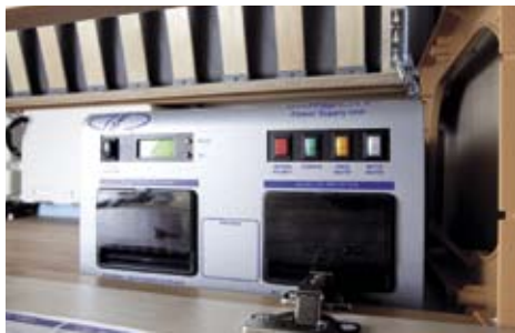
Power switches for mains water and heating are located under the front offside seat. It's not ideal
